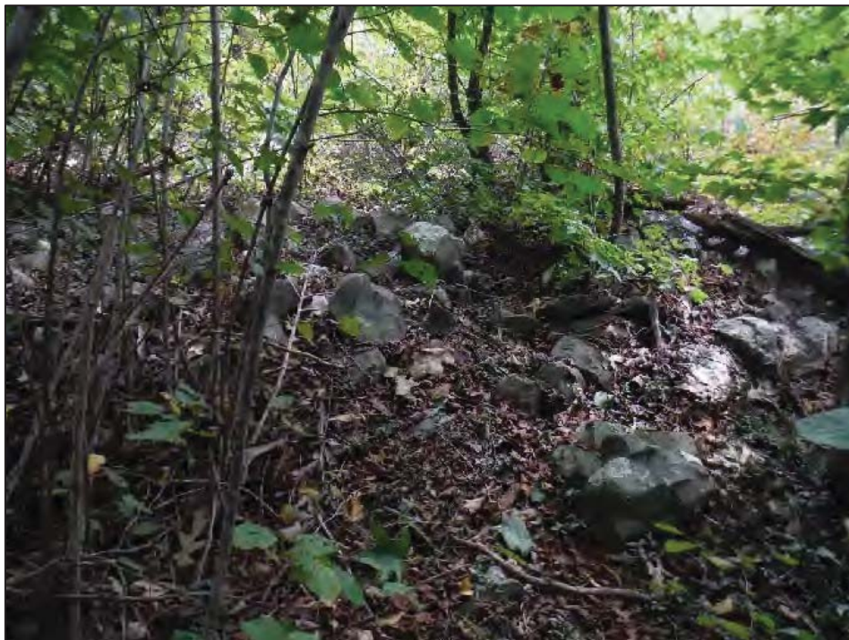
Figure 5.46. Broken down/scattered stone wall around southern portion of 31CH1016**, facing south.
